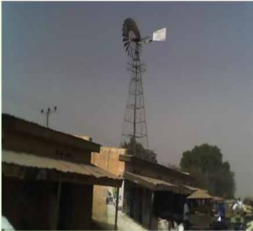
Rehabilitated Windmill for Water Pumping at Kadawa Village, Kano State
